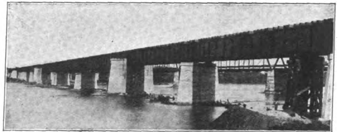
The Completed Deck Plate Girder Structure about 1,550 ft. Long.
